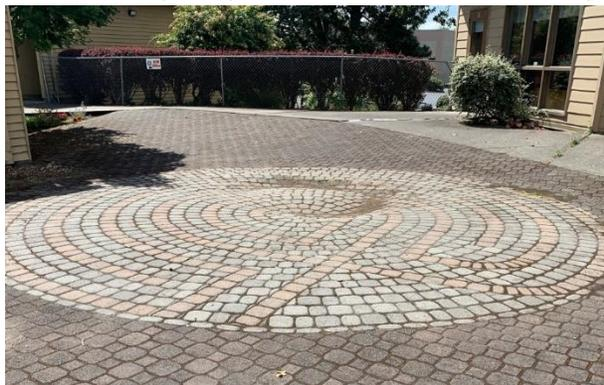
In July 2019, over a four-day period, a small team of volunteers deconstructed the labyrinth to repair it. The team dug up the bricks in the affected area (about 1/3 of the labyrinth area). They carefully removed from each brick the polymorphic sand that had been used during the initial construction.
